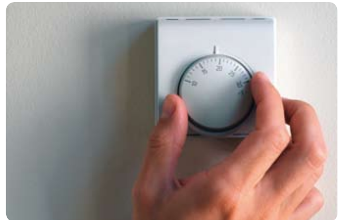
A simple thermostat set at 19°C
